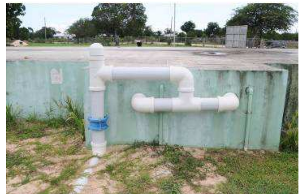
Upflow first-flush diverter (left) and inflow to tanks
