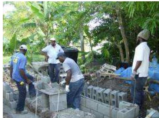
**Figure 9** Construction of the concrete tank platform
