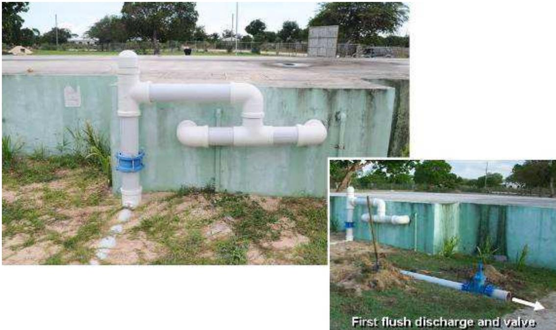
**Figure 17** Upflow first-flush diverter (left) and new inflow pipe configuration to cistern (INSET: discharge pipe from the first-flush)
