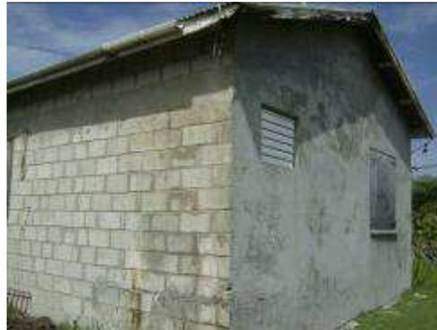
**Figure 11** Demo site before installation (note the rotten fascia board and missing gutter section)
