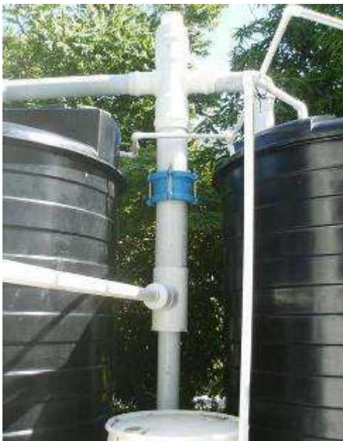
**Figure 10** First-flush diverter and new storage tanks
