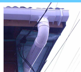
Guttering and downpipe
