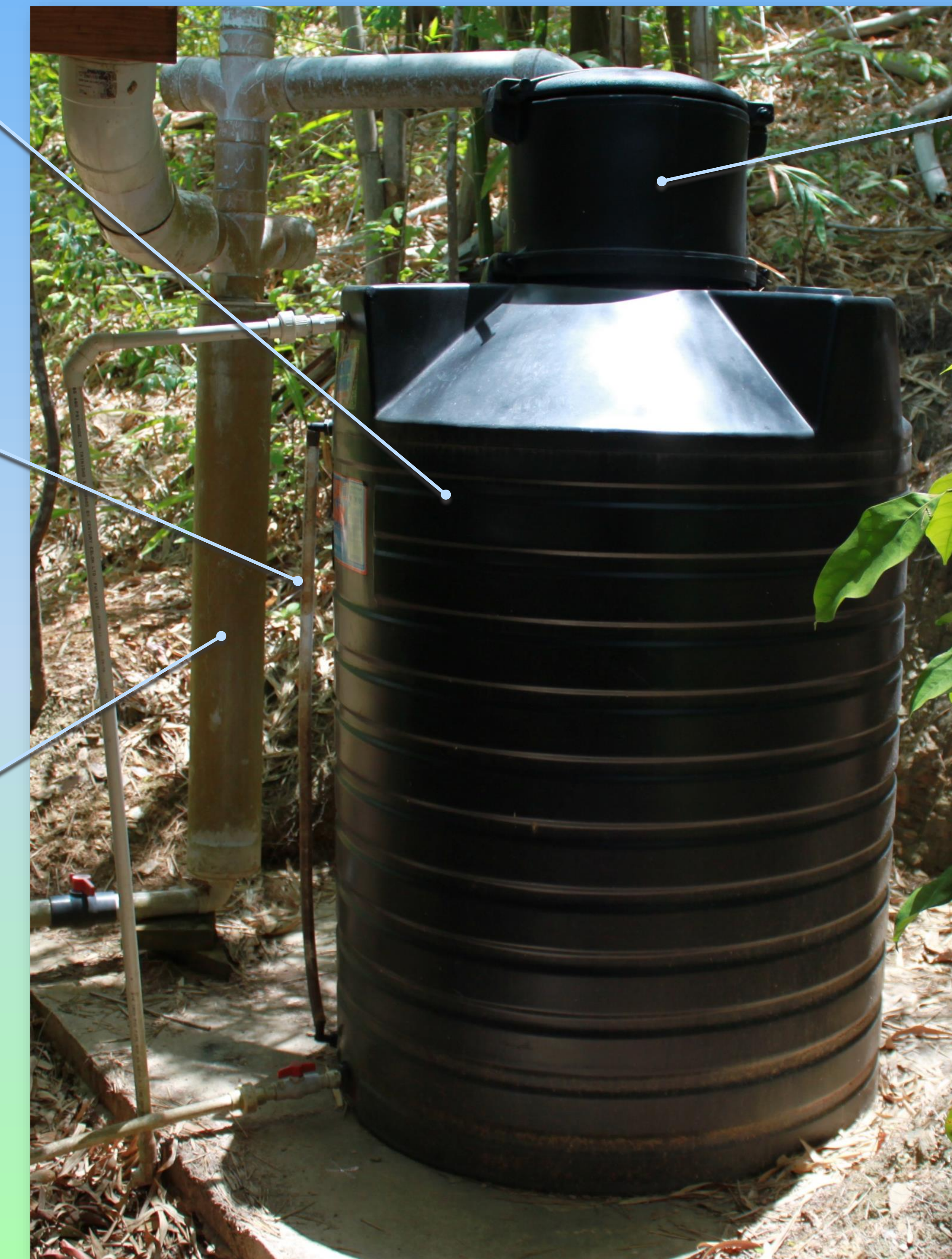
Rainwater Harvesting installation at Fondes Amandes Community Reforestation Project (FACRP) in St. Ann's, Trinidad
